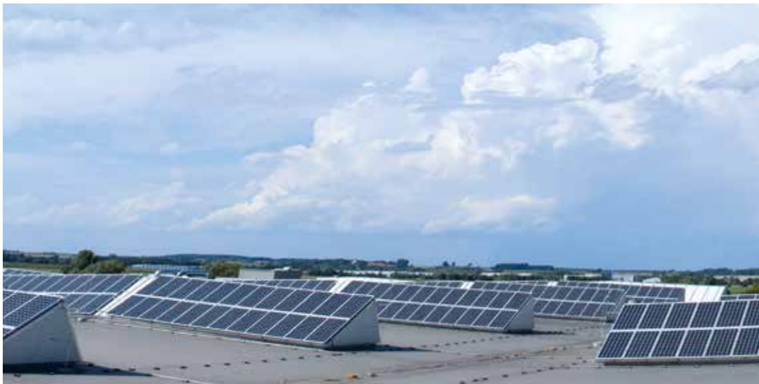
Roof of the production hall of SINGULUS TECHNOLOGIES in Furstenfeldbruck with crystalline solar modules
